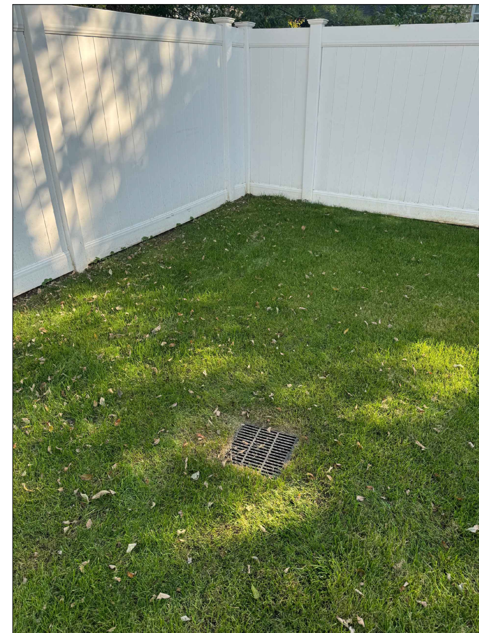
EXISTING PHOTO OF DRYWELL GRATE AT GRADE SCALE: NOT TO SCALE
